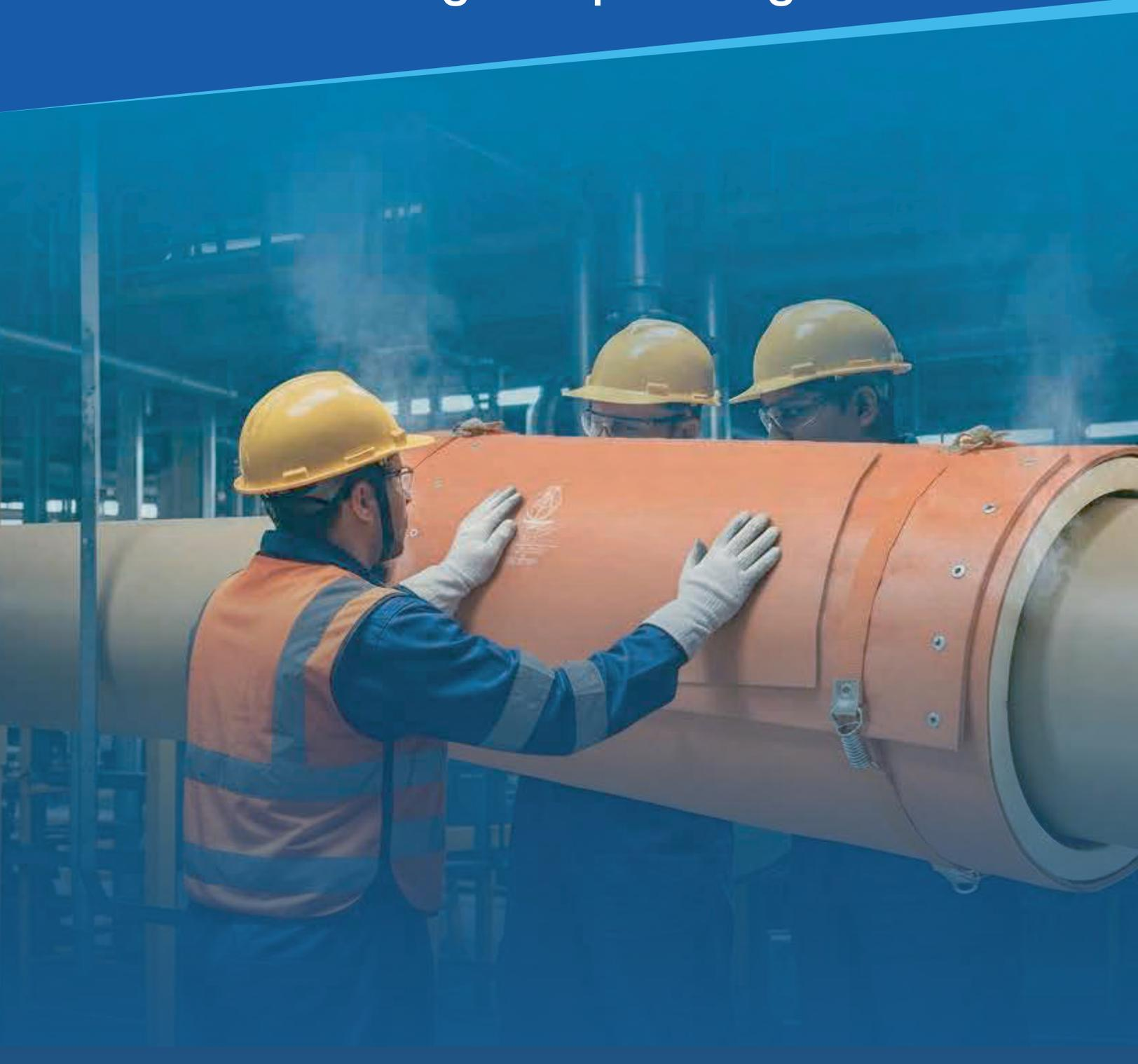
OTA Fiberglass Heating Blankets are engineered for controlled heat curing of adhesive joints and laminated pipe connections in GRE, and RTR piping systems. Designed for harsh field conditions, they ensure uniform temperature distribution, reliable curing, and long-term joint integrity
