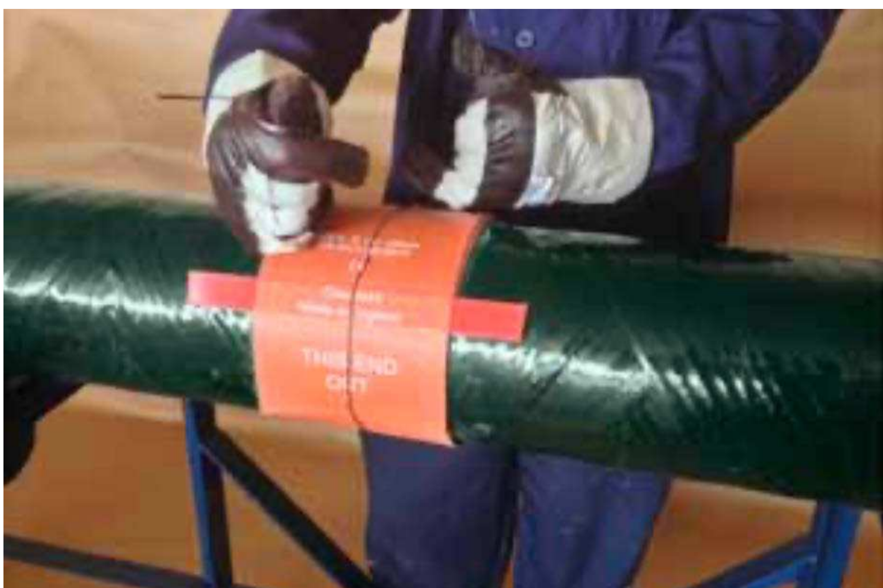
Figure 3.e. Apply Heating Blanket Constant Temp
