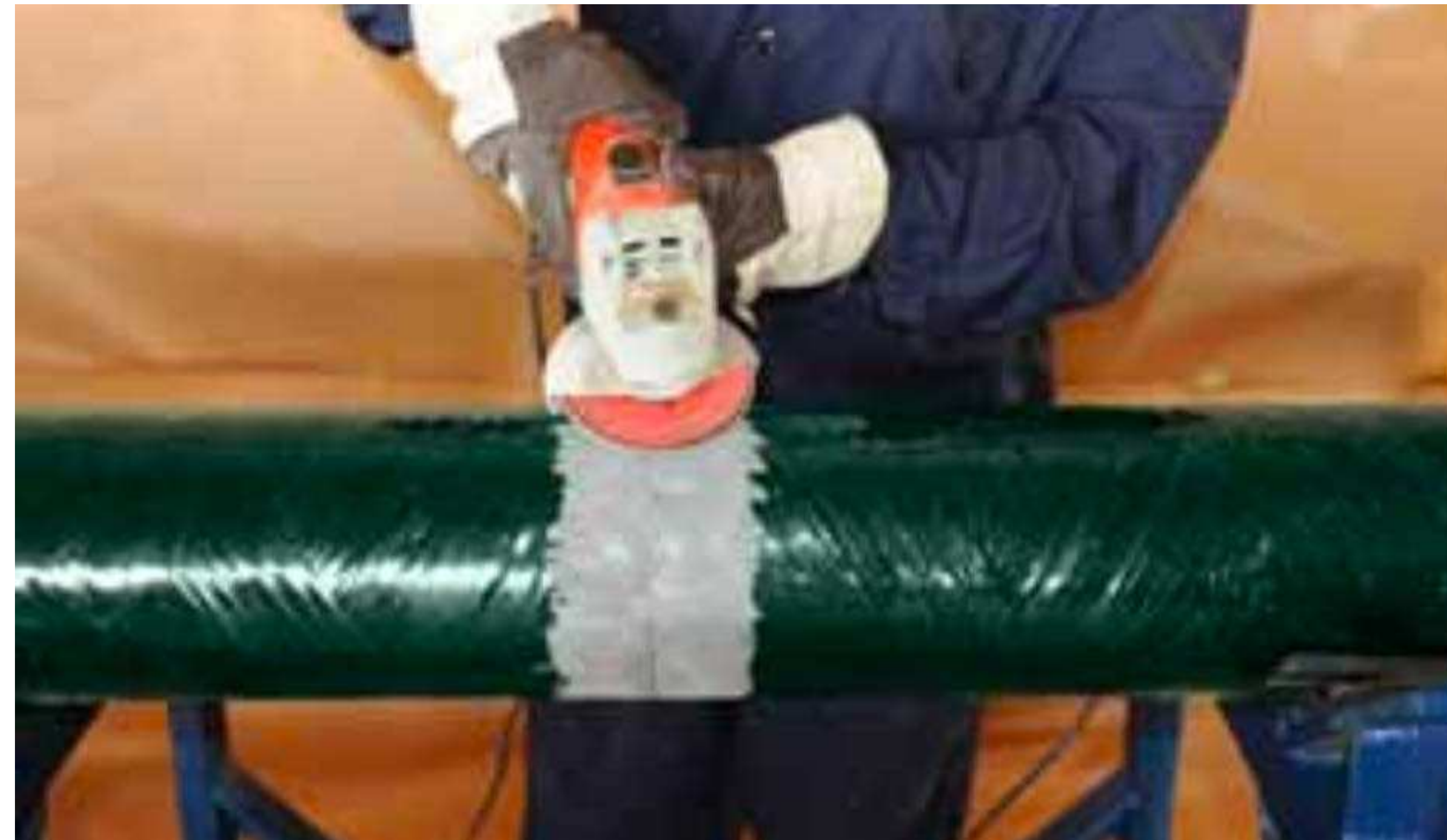
Figure 3.b. Initial Grinding
