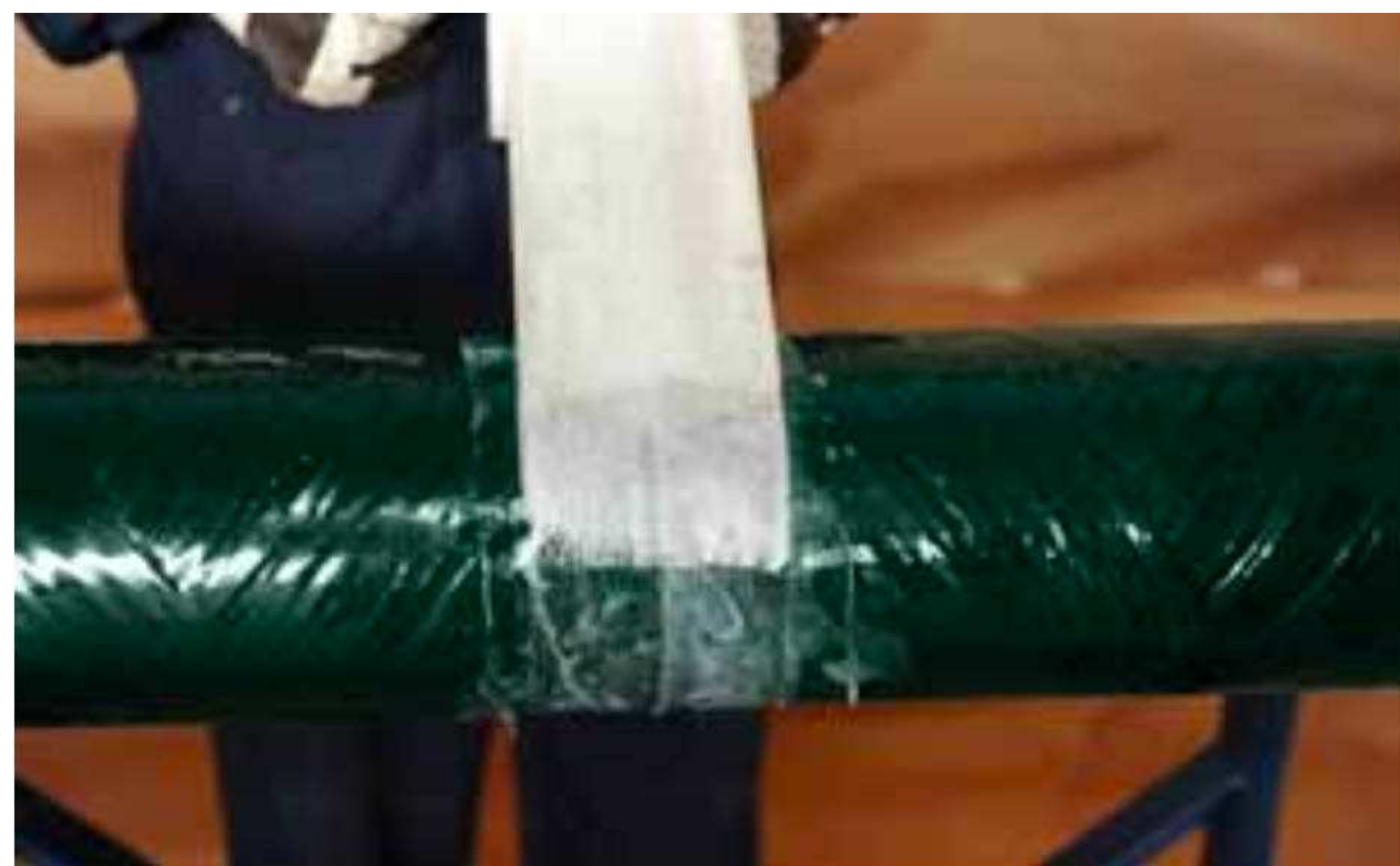
Figure 3.d. Apply WR & CSM Mix
