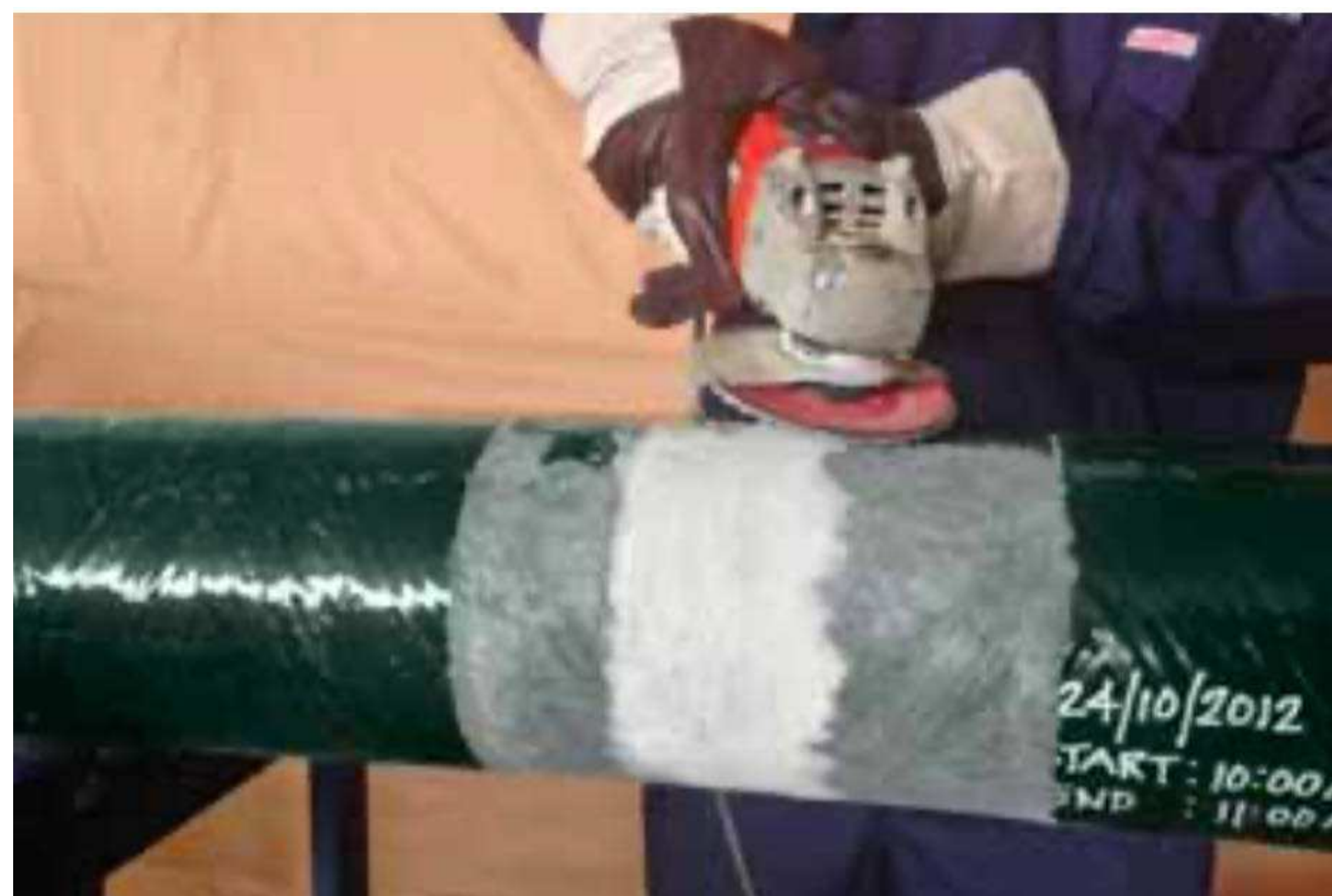
Figure 3.f. Grind surface
