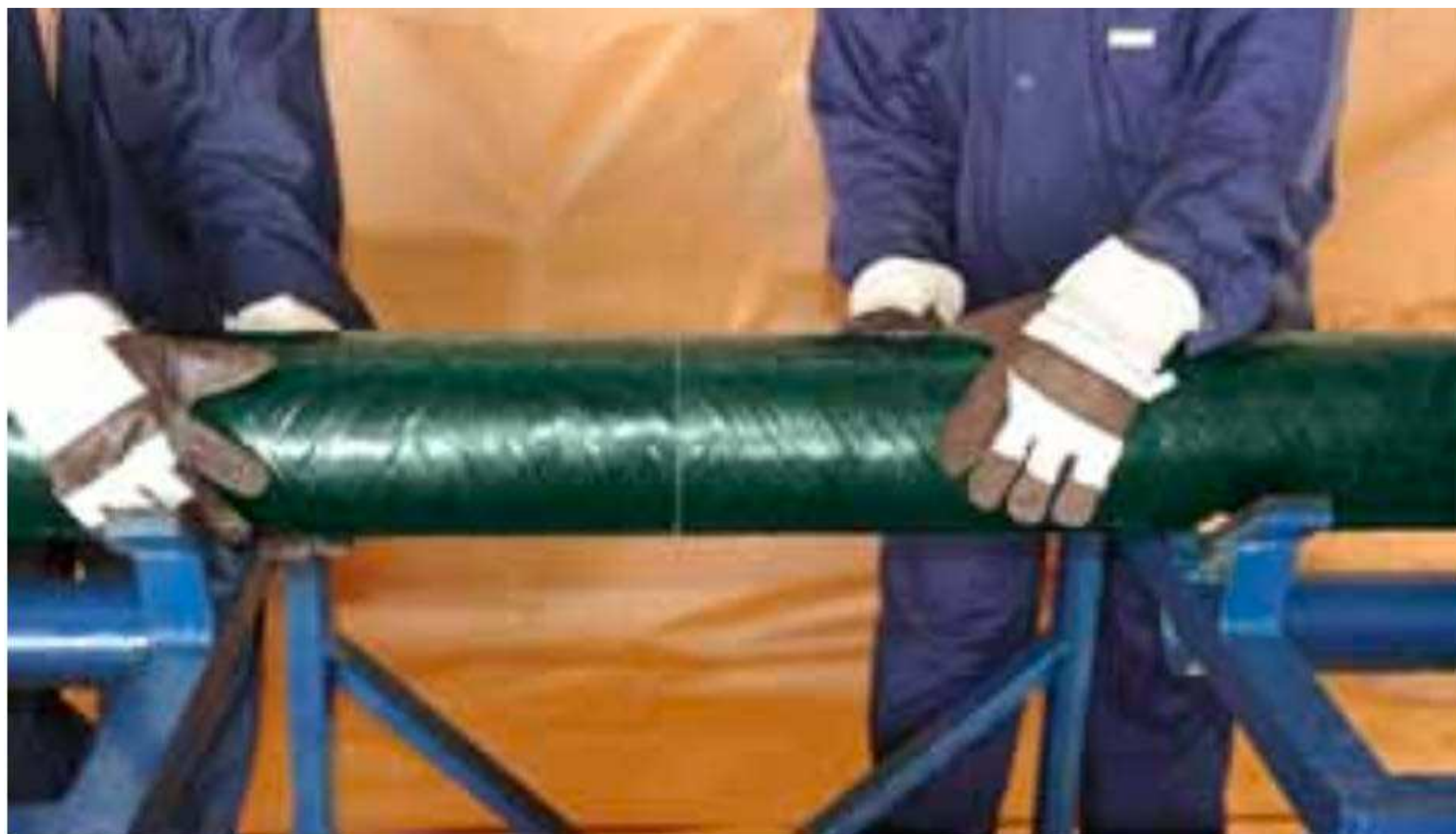
Figure 3.a. Align pipe ends
